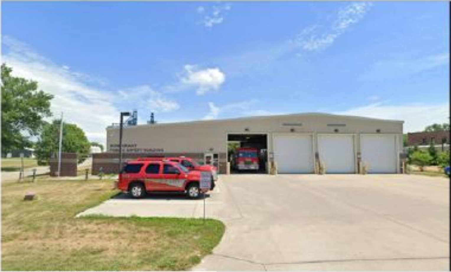
EXISTING WEST FACADE
